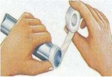
Simply wind the tapes to wrap around male thread of the joint with a right handed rotation. And on each following turn, allow an overlapping of about 10mm
